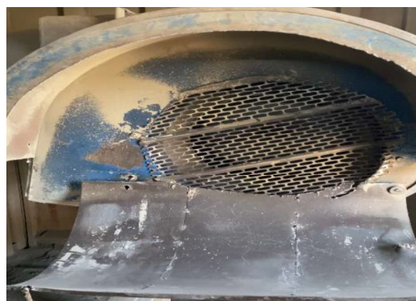
(b) filter cleaning device in the factory
